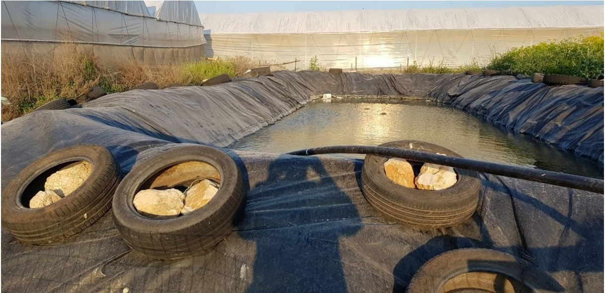
Figure (2): A pond dug in the ground and covered with plastic, the Jericho district.
