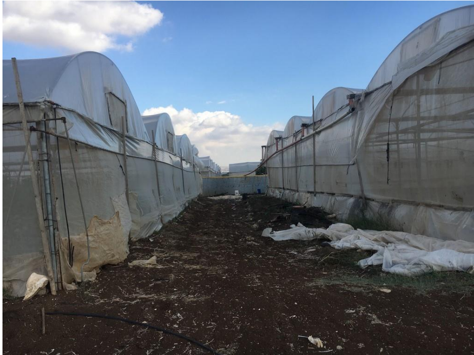
Figure (1): Rainwater is collected by Roofs of greenhouses, the Jenin district.
